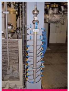
Manifolds for air-pressure services. manufactured by TEG Germany. RK Proball ball valves for general services, from KLINGER Germany.
