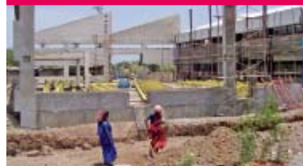
Building extension gasket factory.
