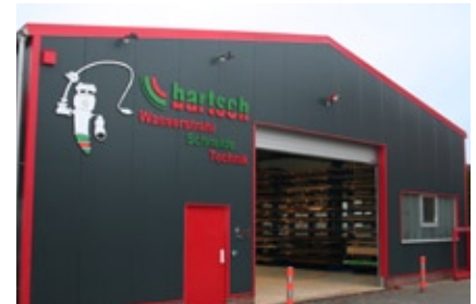
Covering a total area of 400 m 2 , the new hall at BARTSCH GmbH also houses the new water-jet cutting machine. The facade is adorned with Wallenhorster Wasserstrahlschneidetechnik's new «Hoppi» logo.
